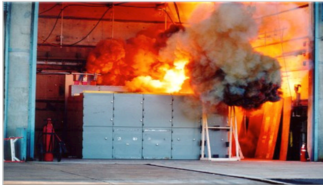
Figure 1 – Unmitigated Arc Fault in an electrical switchboard
