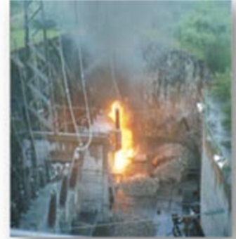
Transformer stations National Power Grid
